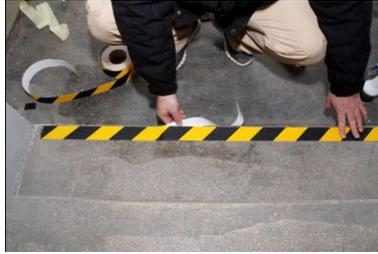
5. Cut tape to necessary length, remove liner partly, angle the tape (keep a distance of 15 mm from the leading edge of stairs to avoid damage of the tapes' edges), take-off the remaining liner and press on the tape.
