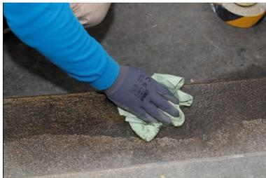
3. Cleaning of the substrate with isopropanol – ventilating is necessary.
