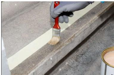
4. Brush blowy, sucking surface with Anti-Slip Primer (in any case when using it outdoor!).
